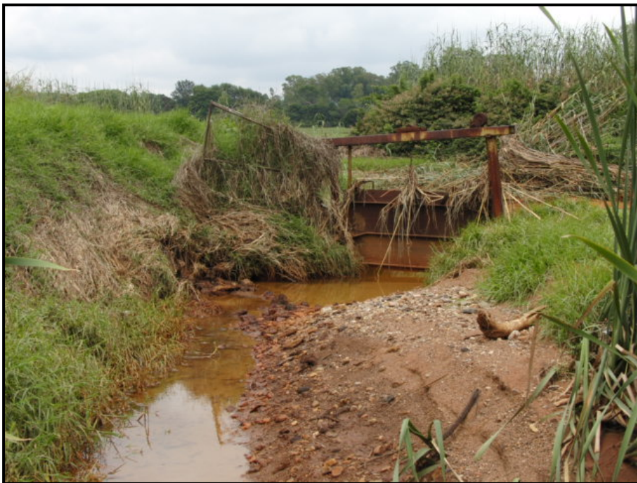
Plate 2. View from downstream of the sluice gate at the entrance to the A-furrow downstream of the Zwartkrans Spring following the high discharge conditions experienced in the Bloubank Spruit in mid-December 2010; note the disruption of flow into the furrow and the sediment deposition on the left bank (right foreground). (Photo: Phil Hobbs).
