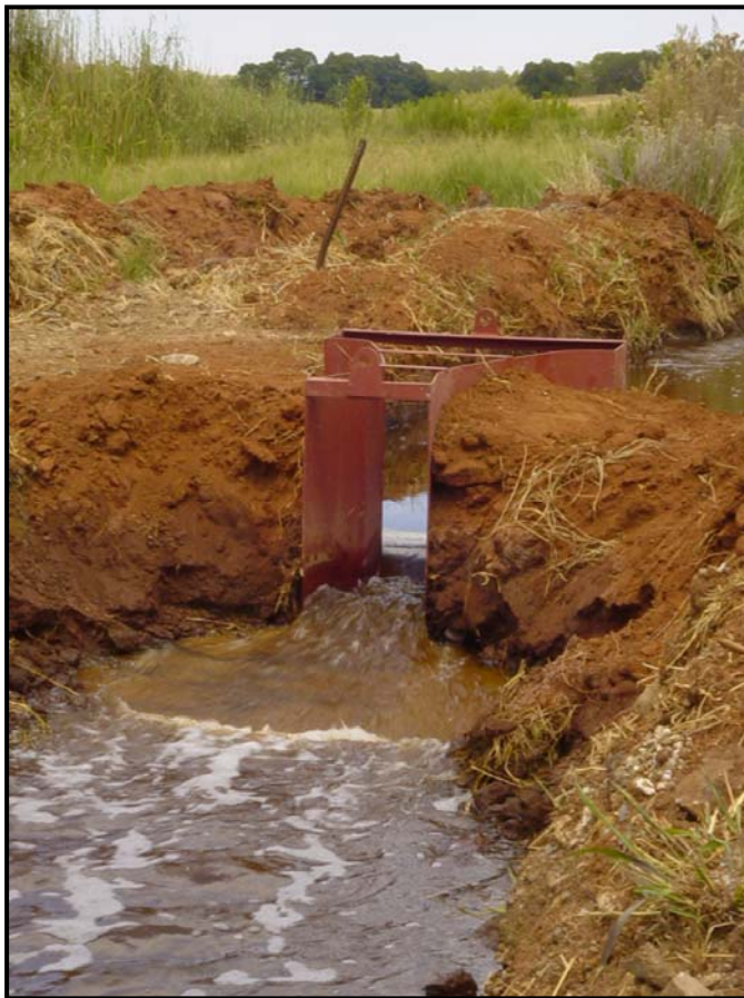
Plate 2. View of the Parshall flume shortly after its installation at the end of the trench draining treated mine water from the Rand Uranium HDS Plant to its point of discharge (end-of-pipe) into the Tweelopie Spruit immediately upstream of the Krugersdorp Game Reserve. This structure was subsequently secured with a concrete abutment to protect the flume from erosion, and also fenced in with razor wire to safeguard the automated water quality monitoring instrumentation installed at this location from theft and/or vandalism. (Photo: Phil Hobbs).
